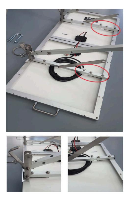
Put the brackets on the edges of the panels, and extend them so they fit (marked red).
