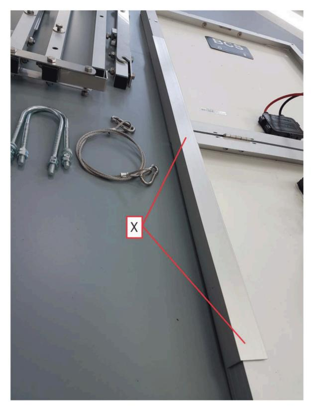
Put the strip (Pos. X) on the side of the solar panels, covering both panels.
